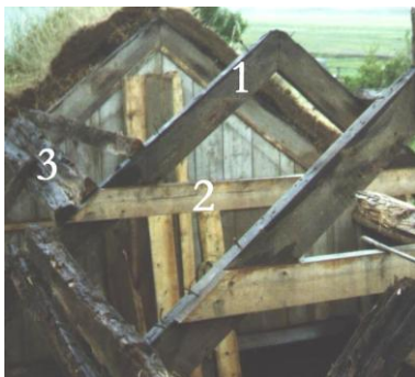
Left. 1 Roof truss, pair of sperrur (rafters). 2 Tie beam. 3 Fragments of wood.
