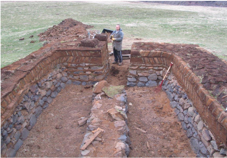
View down into a sheepshed comprising two pens, with a rock manger base between them. Posts supporting the roof beams rested on the rock base. In most livestock sheds in north Iceland from olden times, the walls comprise rock and turf at the bottom, while the upper section of the wall is turf alone.
