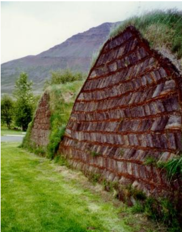
Gable walls of Nýi-Bær at Hólar, built of klömbruhnaus.
