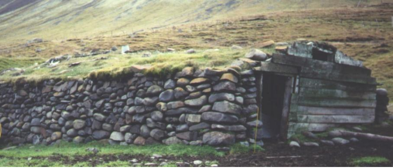
This sheepshed at Skatastaðir is built of scree rock, with strengur turf strips (in the wall). The shed has a manger along one of the long walls. Shallow-pitched pairs of rafters rested on flat rocks atop the walls.
