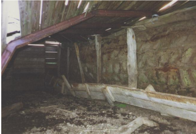
A cow-barn wall at Halldórsstaðir made out of clamped blocks and strips . The stalls were opposite this wall, and protected it. The far wall, to more than halfway up, was made of stone with strips between the courses.
