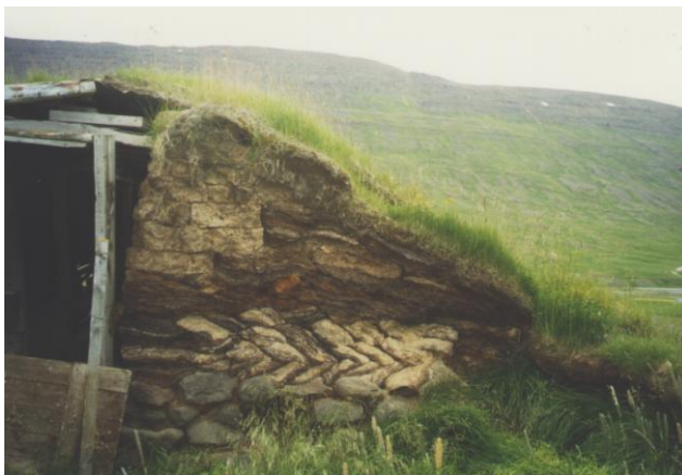
In the gable of the sheep barn at Hof in Hjaltadalur you can see milk-pen blocks that are lying flat, at the top, and set overlapping each other below. At the bottom of the wall are stones. The barn is roofed over with grass sod turf.
