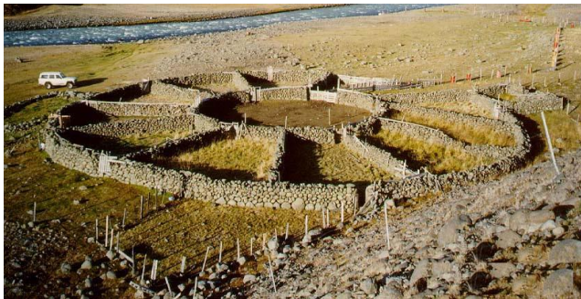
This old sheep corral at Bjarnastaðahlíð in Vesturdalur, called Hlíðar-rétt, is completely made of stones from the river-bank around it. This sheep corral is still in use, every fall. Structures made of stone, without turf can be seen in many places around the country.
